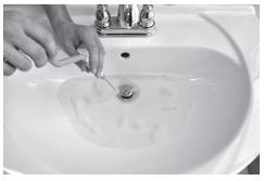
**2)** Place one hand on the sleeve. Using the other hand, rotate handle 360 degrees several times or until the first signs of resistance are felt. Do NOT force rotation.
