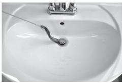
**3)** Carefully pull snake and debris from the drain. Remove wand from reusable handle (see above) and discard along with drain waste.
